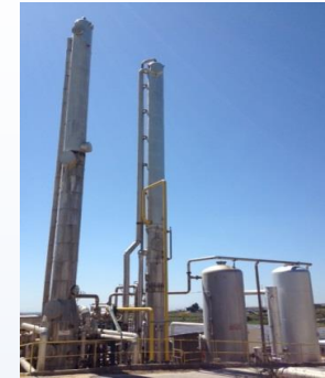
CO 2 removal plant based on Giammarco-Vetrocoke Process – Ragusa (Italy)
